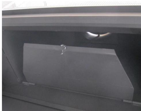
The angle of the damper must be adjusted in such a way that no smoke is kicked back into the living room. The smaller the angle of the damper, the better the heat emission towards the room, but the more difficult it is to evacuate the flue gasses through the flue gas duct, and the greater the risk of smoke being kicked back.
